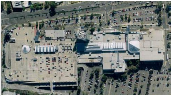
Project Aspect: Flat Deck Roof Structure – MAXIMUM SOLAR ABSORPTION
